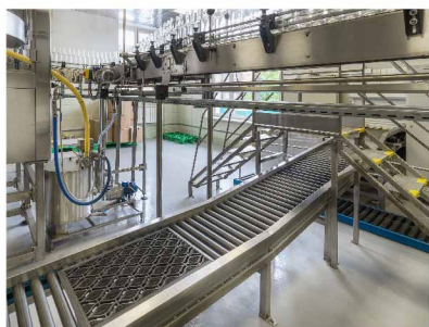
STRUCTURAL TUBES FOR CONVEYOR
